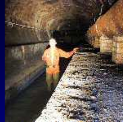
a sewer in Paris
